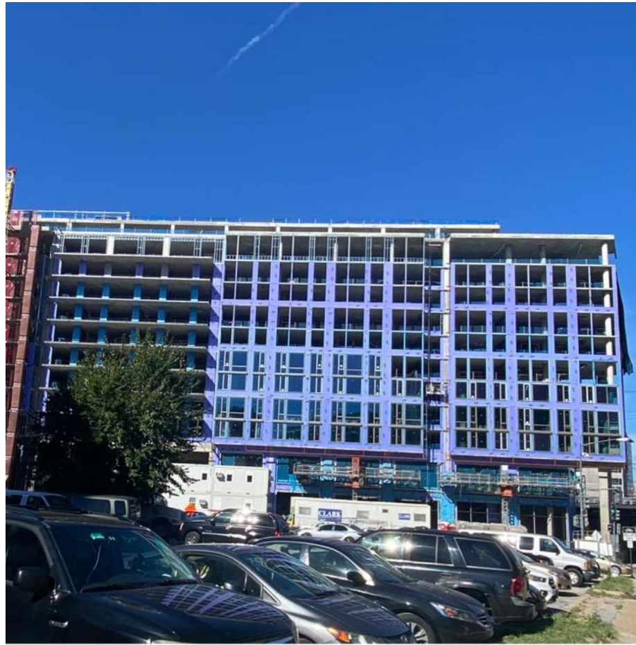
1. 1200 Third St NE_ 12 Floors Plus Penthouse
