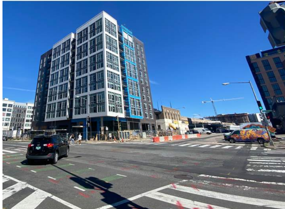
4. 5th St NE & Florida Ave NE_ 12 Floors
