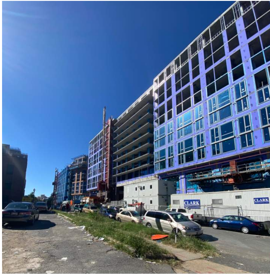
7. 1200 Third St NE_ 12 Floors Plus Penthouse
